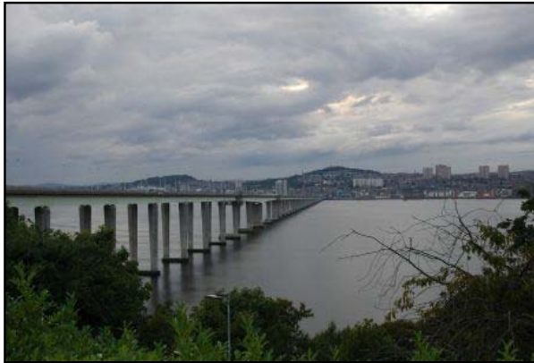
Tay Road Bridge, Dundee
