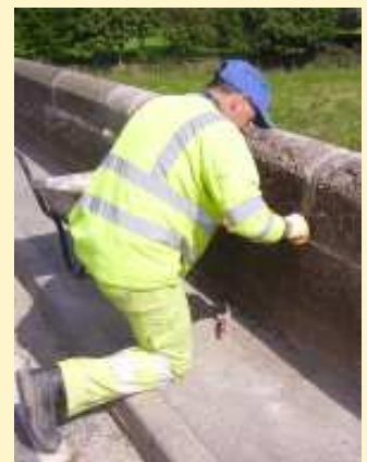
Alan Findlay puts last stone in place
